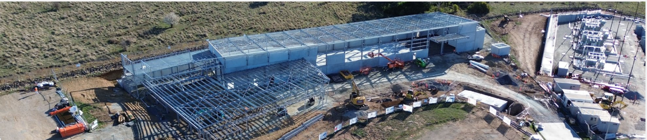
CONSTRUCTION OF SAMSARA ECO'S R&D FACILITY.
